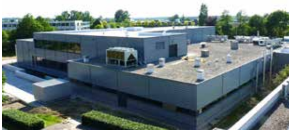
Donaldson European Technical Center. Expanded testing capabilities for engine filtration businesses in October, 2010.
